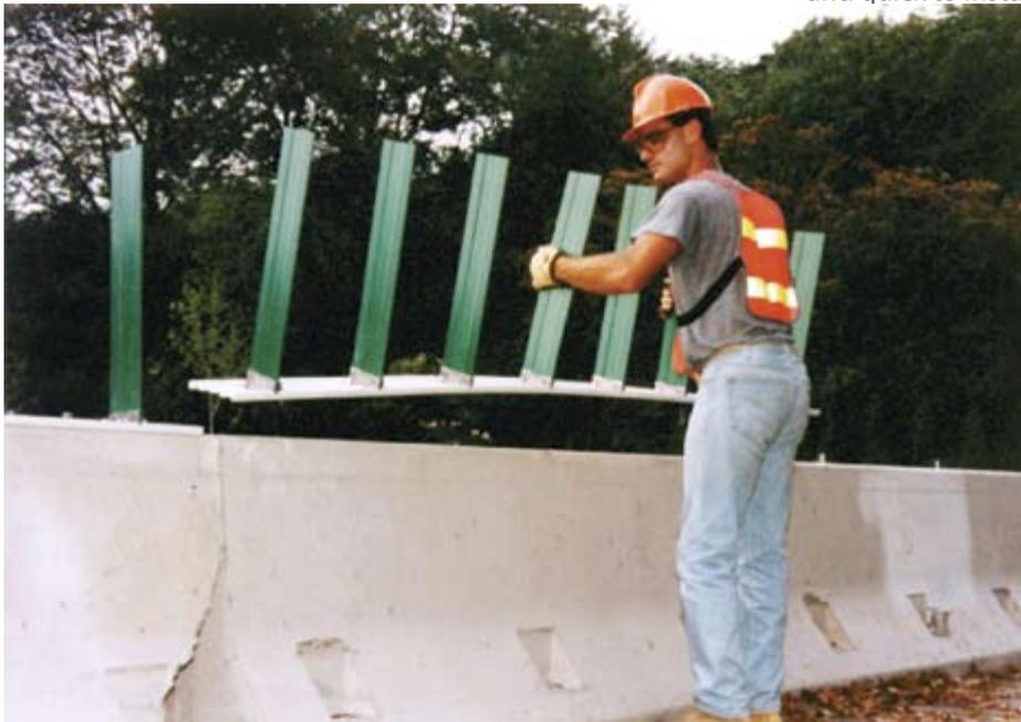
Carsonite's MGS allows the modules' blade angle to be changed as needed, without disassembly or removal from the barrier. For permanent installation use model NMGS or for work zone applications use model WMGS). The Carsonite WorkZone Modular Guidance System® features a narrower rail base (3" vs 6", nominal) and adhesive-set threaded anchoring inserts for bolting the modules to the concrete barrier. Each product comes in 10', 12', 12½', and 15' lengths.
